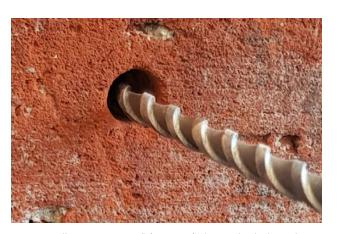
Drill an approx. 10" (250mm) deep pilot hole with a 6mm diameter PYTHON masonry drill bit and rotary only drill.
