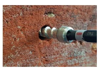
**04** Install the PYTHON C using a TORX T40 bit and impact driver.
