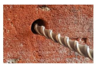
O2 Drill an approx. 250mm deep pilot hole with a 6mm diameter masonry drill bit.
