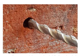
To countersink the screw head, drill a 7mm deep hole with a 10mm diameter masonry drill bit.
