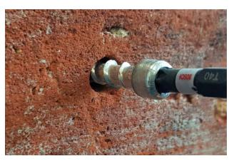
Install the PYTHON C using a TORX T40 bit and impact driver.
