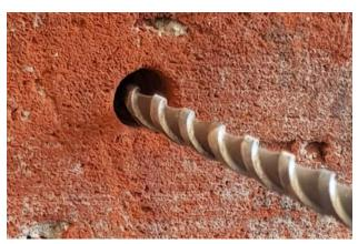
O2 Drill an approx. 250mm deep pilot hole with a 6mm diameter masonry drill bit.
