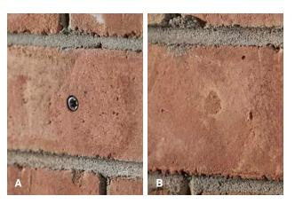
A. Leave head exposed. Or;B. Cover head with colour matched putty as per architectural specification.
